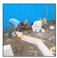
**Screens and decks:** Screens were created using 75x75mm H4 treated pine posts set in rapidset concrete with blueboard panels fixed with masonry nails and then painted.
